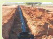
Under Ground Drains
